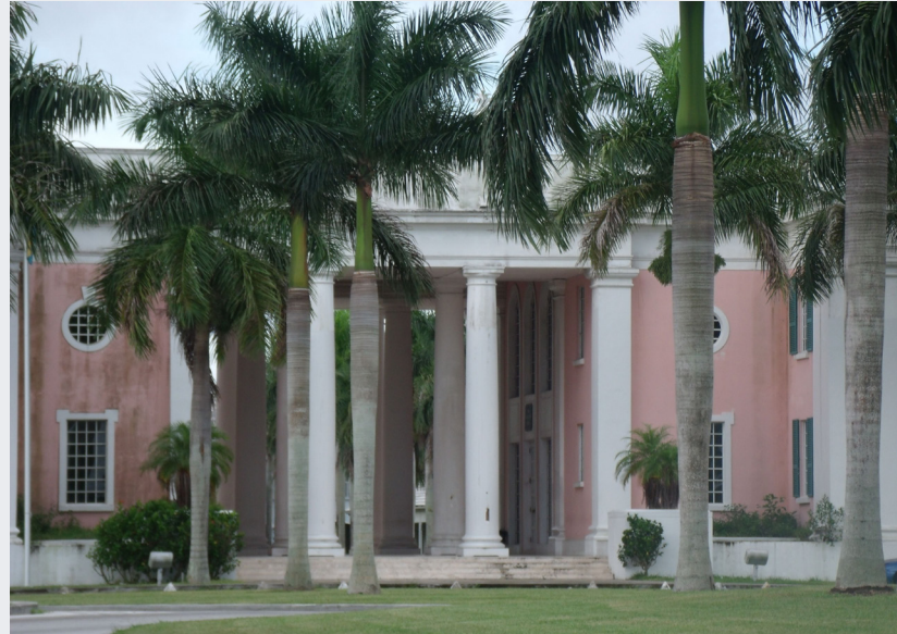
Garnet Levarity Building, Supreme Court Freeport, Grand Bahama.
